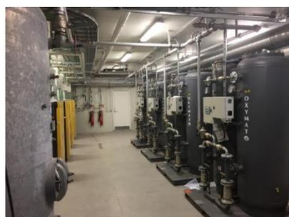
produced by an Oxymat PSA generator. The PSA installation has not only increased the number of smolt being produced on land, but it has also increased the size of
